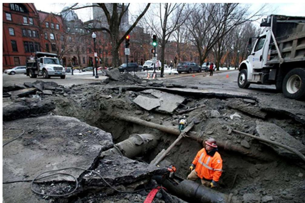
**Figure 2-2: An example of the damage caused to other community assets following the break of a relatively small Trunk Water Main. This damage has the potential to render other community infrastructure unusable until repairs are effected.**
