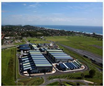
The Gold Coast Desalination Plant uses reverse osmosis to turn seawater into drinking water - a climate-resilient supply of water during drought.
