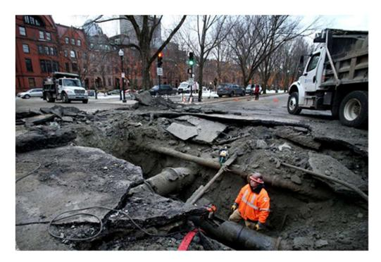
Figure 2-2: An example of the damage caused to other community assets following the break of a relatively small Trunk Water Main. This damage has the potential to render other community infrastructure unusable until repairs are effected.
