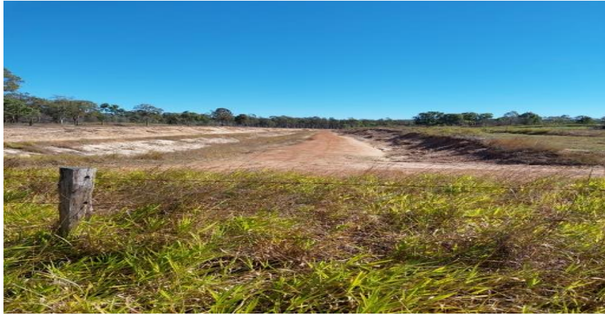
Figure 4: Clarendon Channel Berm Maintenance
