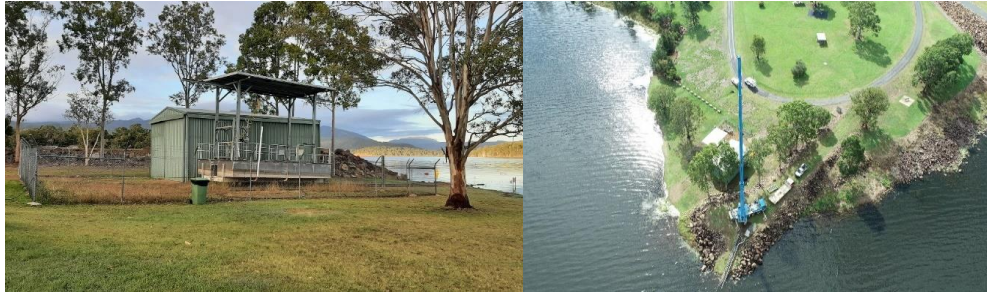
Figure 4: Bromelton Weir before, during and after the project.
