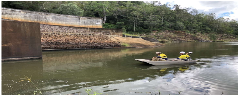
Figure 5: 5 Yearly Inspection continued –crossing Yabba Creek.
