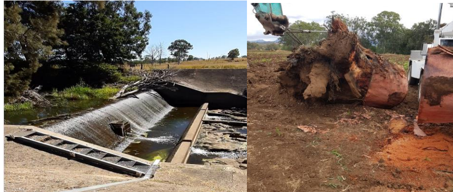
Figure 5: Aratula Weir –Before and after photographs are below.
