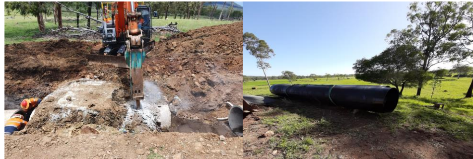
Figure 4: Upper Warrill pipe line breakages works.
