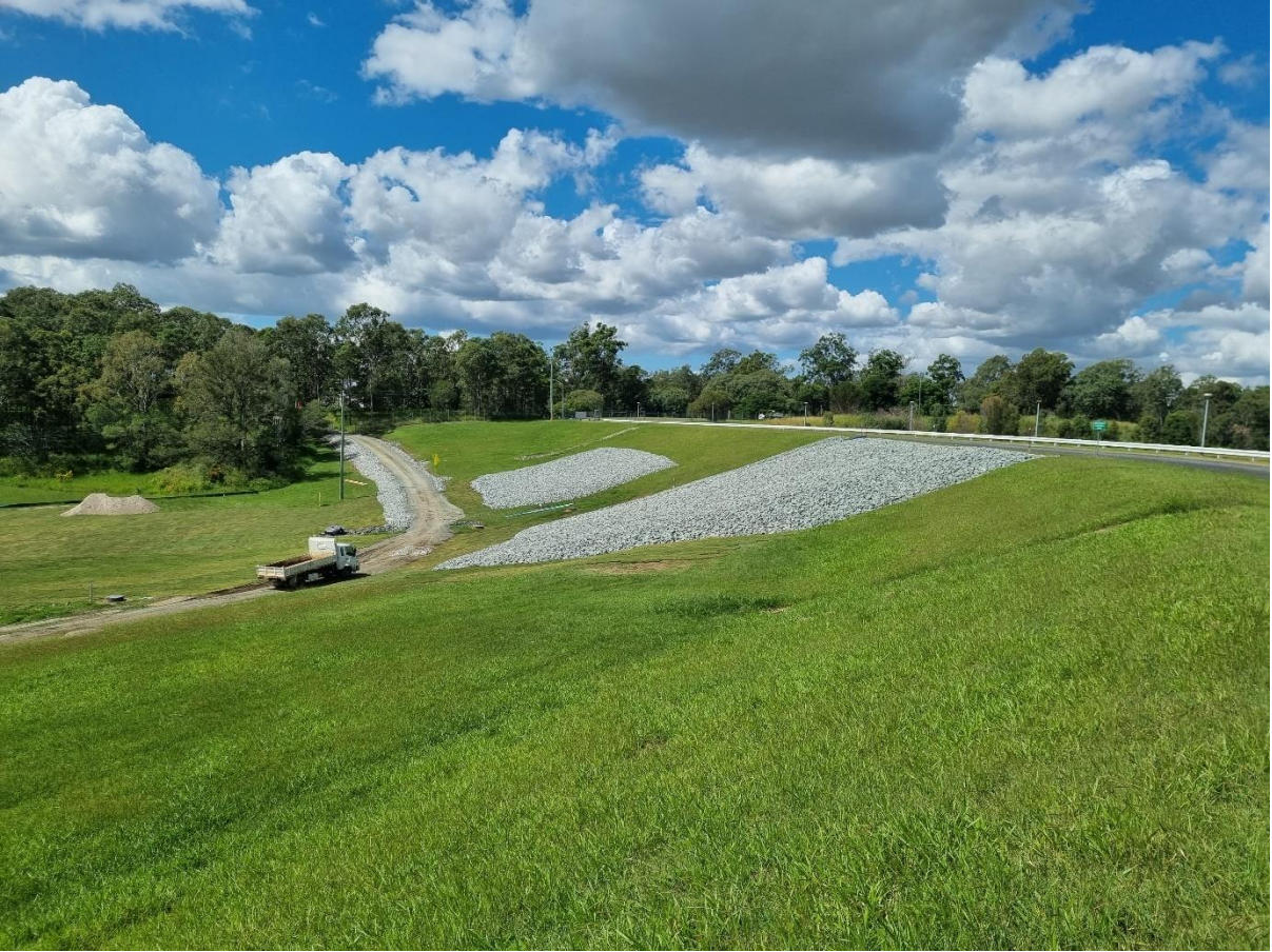
COMPLETED FILTER BUTTRESS
