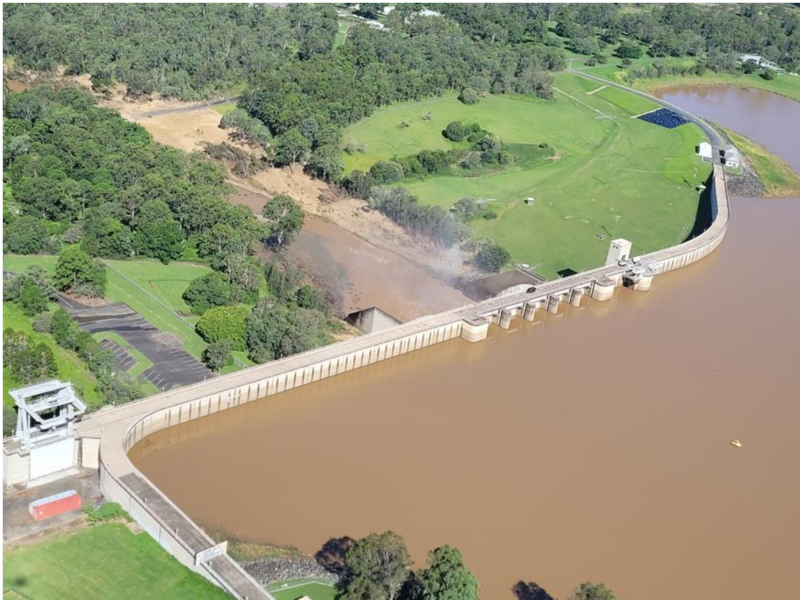
NORTH PINE DAM – MARCH 2022
