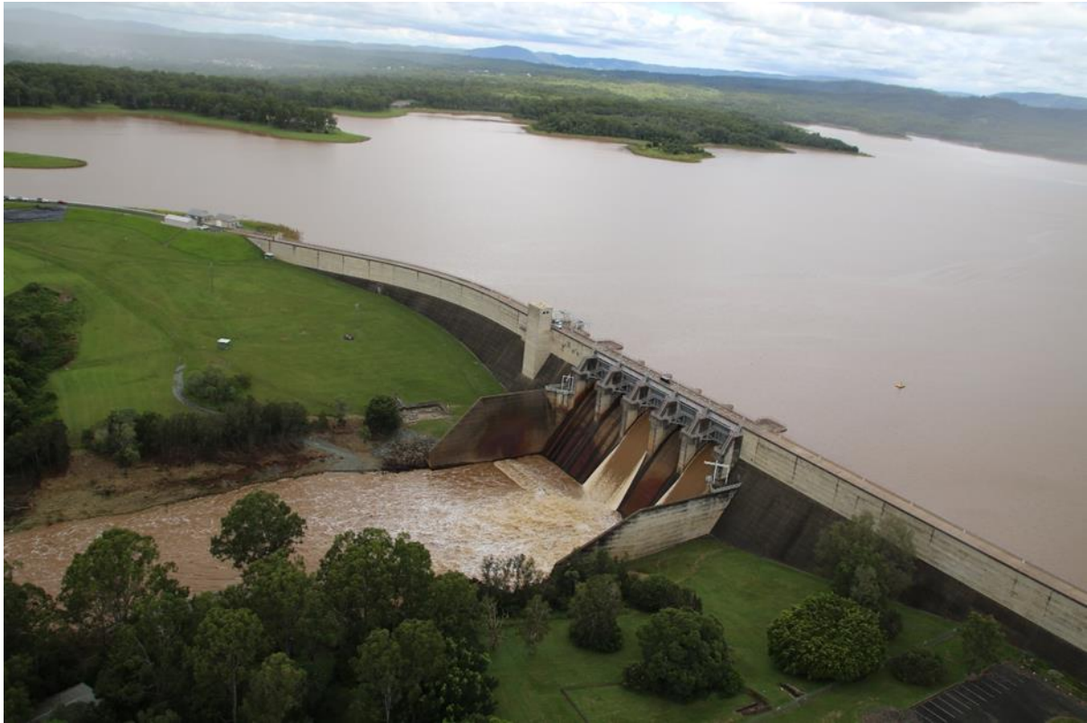
NORTH PINE DAM MAIN DAM CONCRETE EMBANKMENT – MARCH 2022
