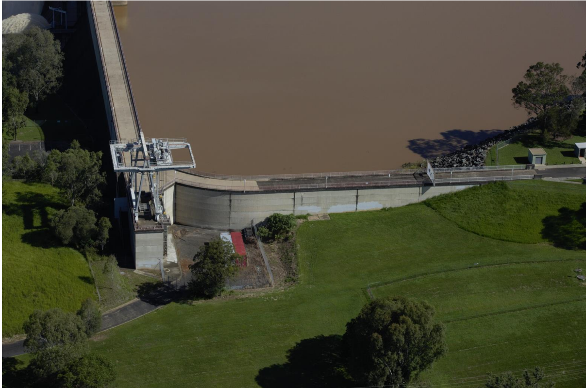
LEFT BANK EARTH/ROCK SHOULDER EMBANKMENT
