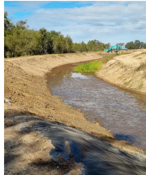
Figure 6: Post flood cleaning and repair works on Brightview Channel
