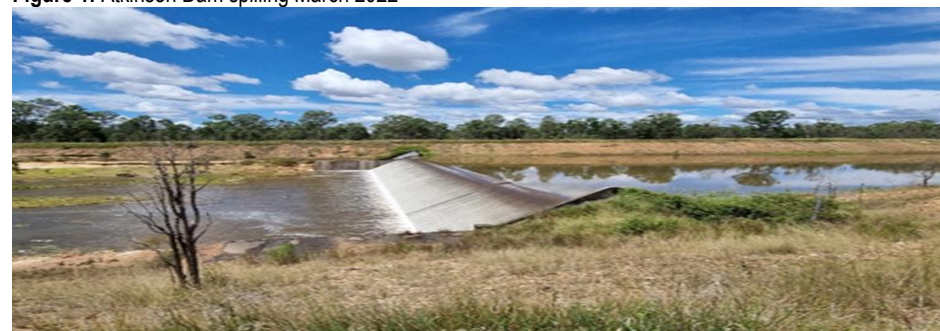
Figure 1: Atkinson Dam spilling March 2022
