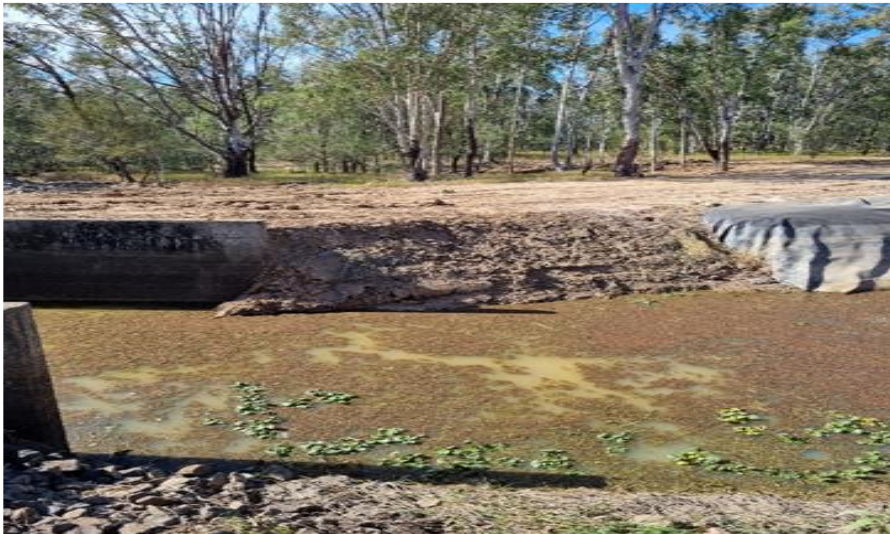
Figure 5: Repair works on washout Brightview Channel
