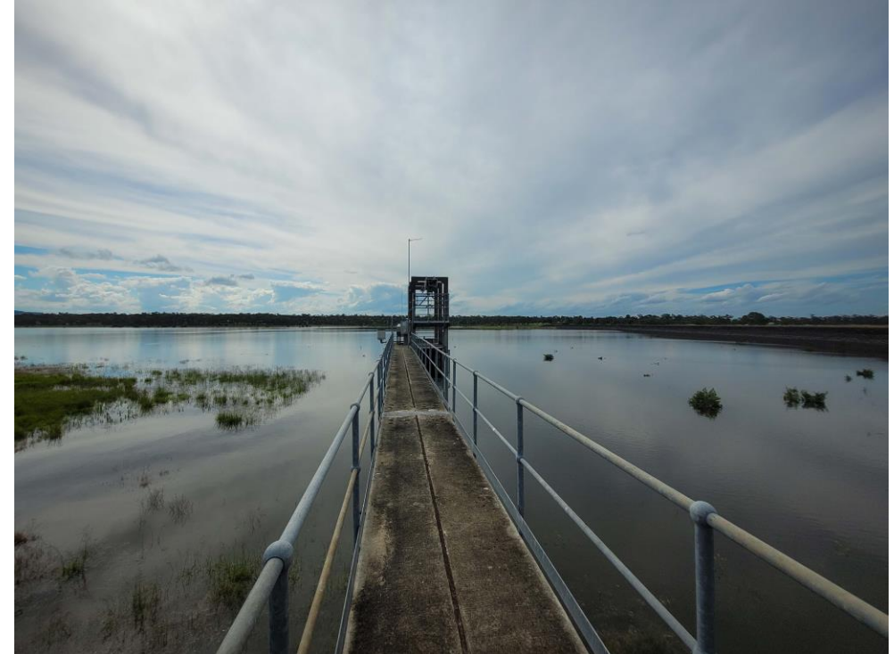
Figure 6: Bill Gunn Dam Intake Tower
