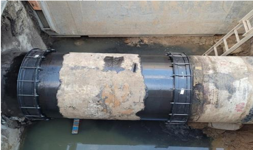
Figure 4: Bill Gunn inlet/outlet pipe repair
