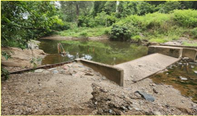
Figure 4: Borumba Weir (Measuring) after clean.
