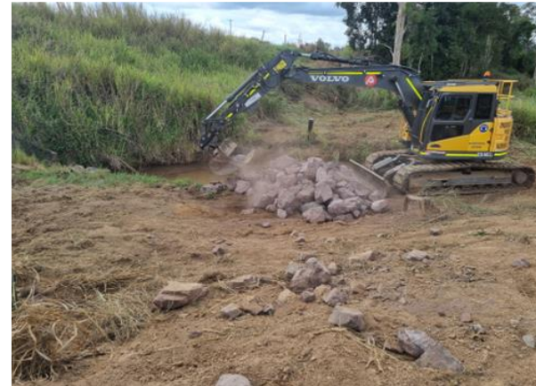
Figure 10: Repairing cross drains – Pie Creek
