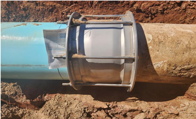
Figure 9: Emergency repair to Pie Creek pipeline
