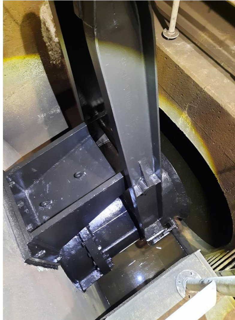
Figure 4.1: Maroon Cone Valves painting completed
