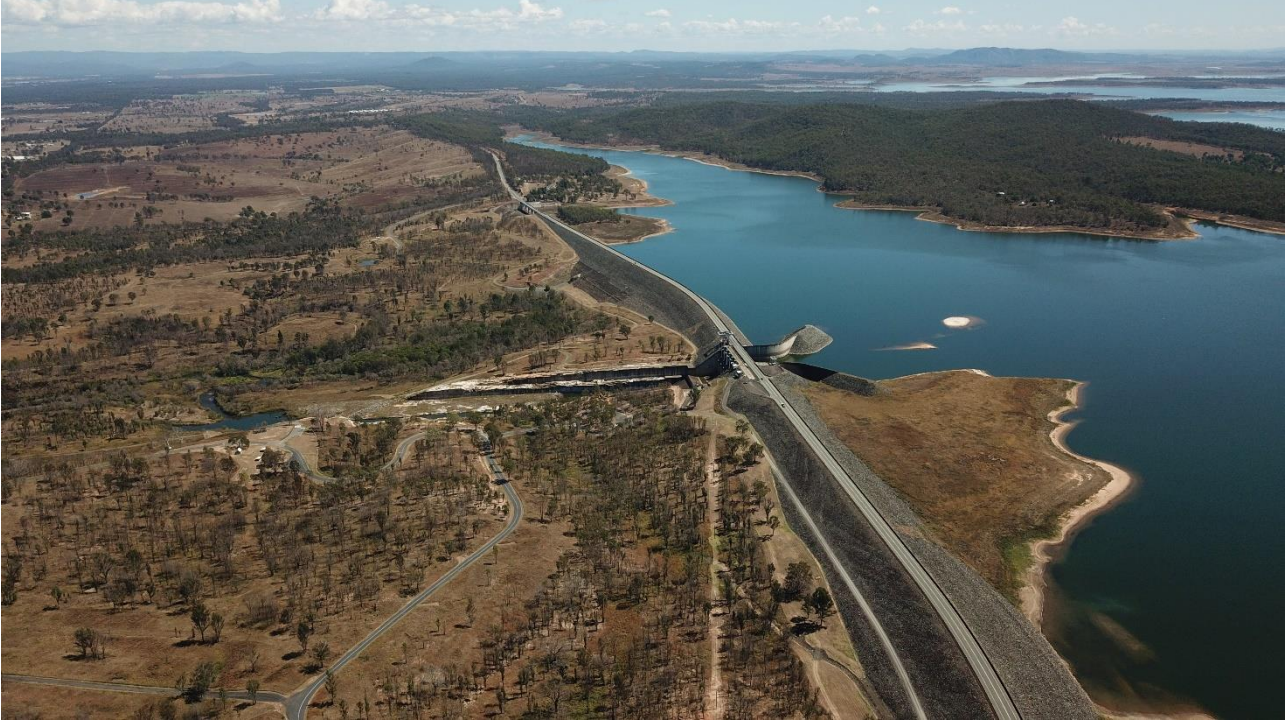
Figure D.1 Wivenhoe Dam Aerial View
