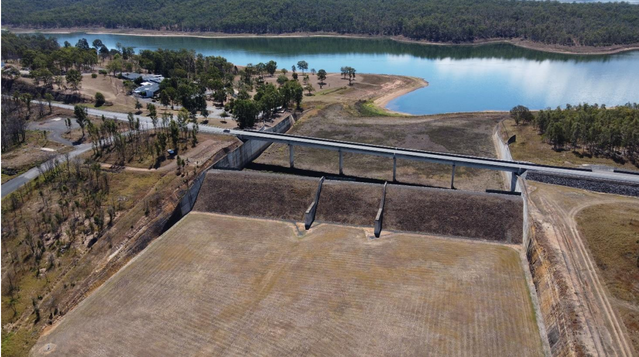
Figure D.3 Wivenhoe Fuse Plugs (looking upstream)
