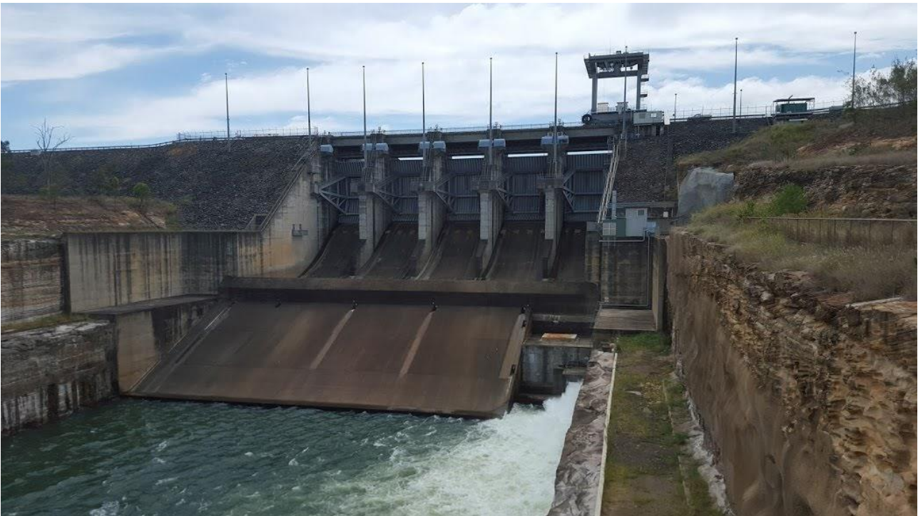
Figure D.2 Wivenhoe Dam Main Spillway (looking upstream)
