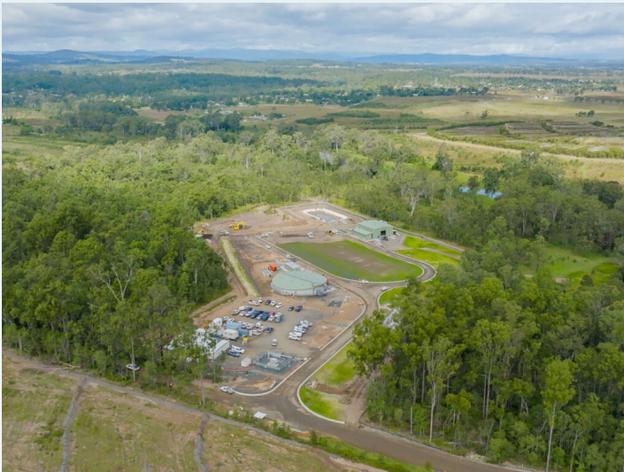
South West Pipeline Wyaralong Transfer Station - aerial view
