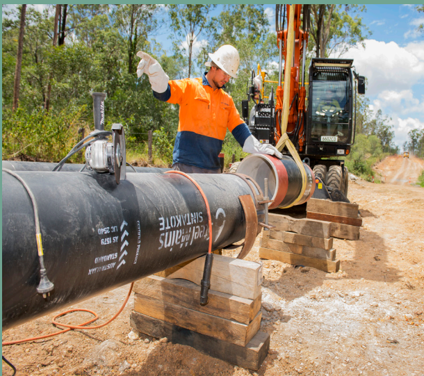
Pipeline worker and section of South West Pipeline
