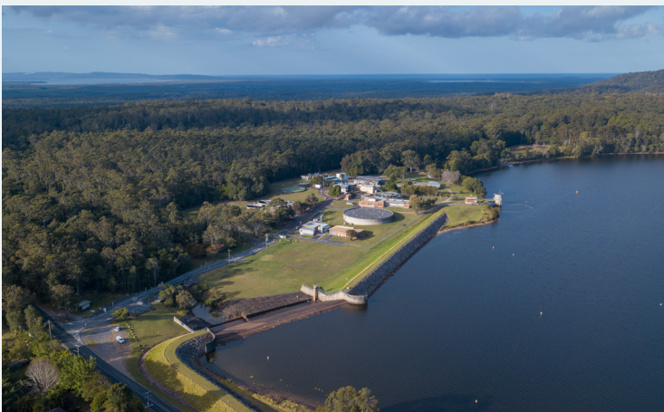
Noosa Water Treatment Plant and existing dam wall at Lake Macdonald
