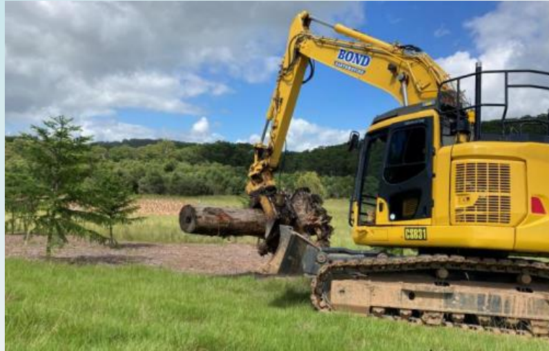
Excavator placing root balls to build habitat stack.
