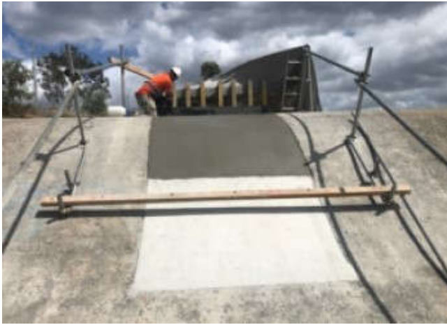
Image(L): Reinstating the slot in the spillway
