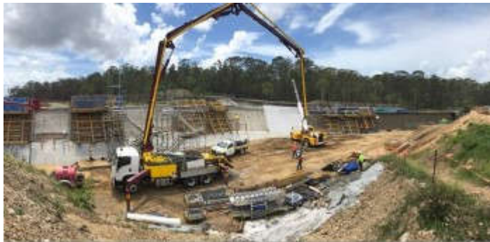
Image: Concrete work on the spillway
