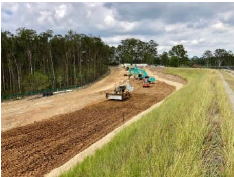
Image: Earth embankment under construction
