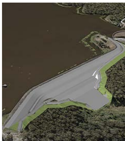
Image: Embankment post upgrade
