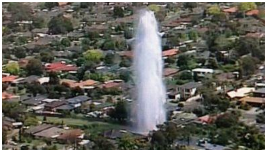
Figure 4 – A Burst Trunk Water Main in Melbourne in 2012 sent water jets 80 m into the air with 2 million litres of water released. Neighbouring roofs collapsed and extensive property and cars were damaged as a result.
