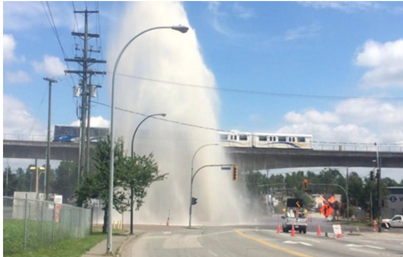
Figure 2 – Due to the very high pressure at which Trunk Water Mains operate, a break has the potential to release dangerous water jets.
