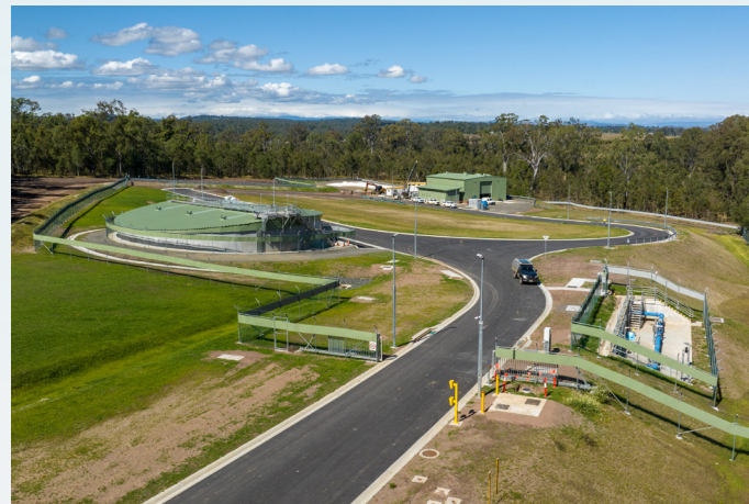
South West Pipeline Wyaralong Transfer Station
