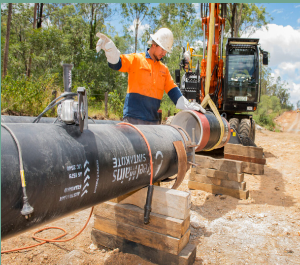
Pipeline worker and section of South West Pipeline during construction
