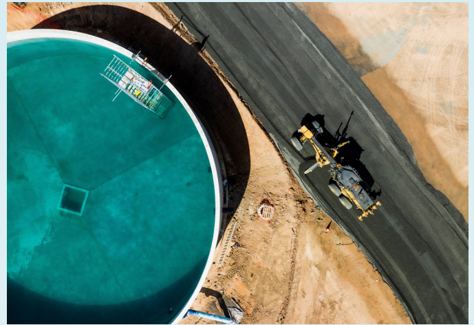
Construction of the South West Pipeline Wyaralong Transfer Station
