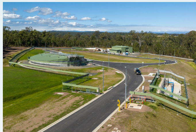
South West Pipeline Wyaralong Transfer Station
