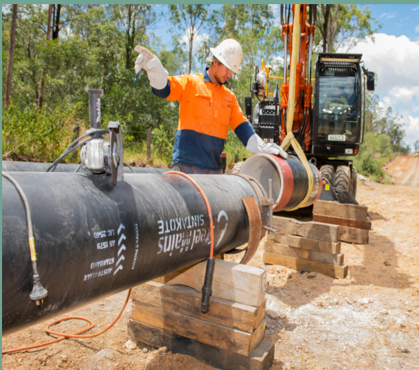
Pipeline worker and section of South West Pipeline during construction
